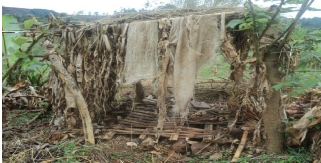
Photo 2. Household pit latrine with superstructure and roof that needs maintenance in rural community of selected Sub districts ( Kebeles ) in Chencha district, February 2013
